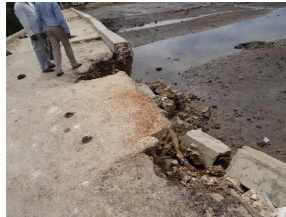
The sea wall at Siyu village
